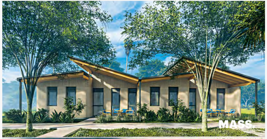
Mvule Gardens in Kenya, Africa's largest 3D-printed affordable housing complex is built with TectorPrint
