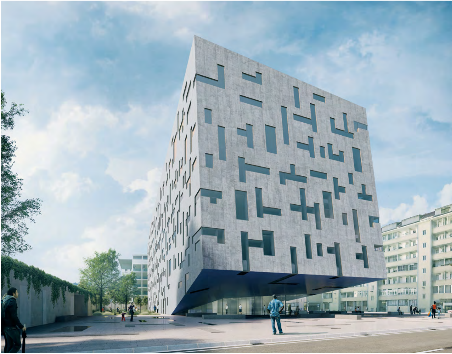
New CAP Group Headquarters, Milan, is built with ECOPact green concrete with 35% lower CO 2 to achieve LEED Gold certification
